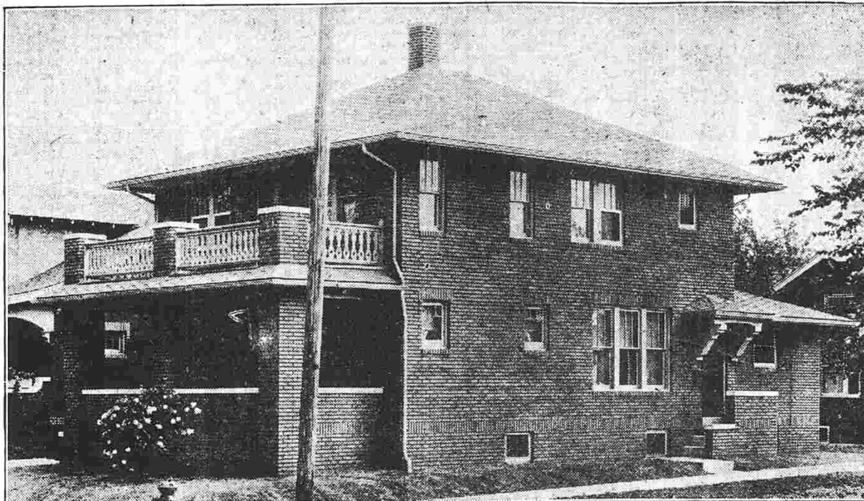
This handsome brick veneered house grew from an old frame structure. This view is evidence of the possibilities of modernization.
